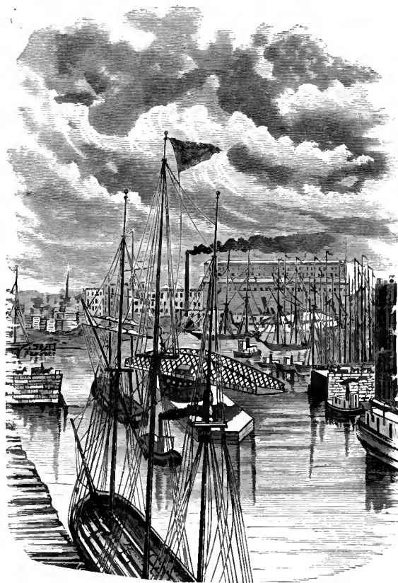
CHICAGO RIVER—CLARK STREET BRIDGE.
